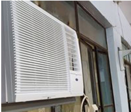
HCC started installing the air-conditioning units in the classrooms.
